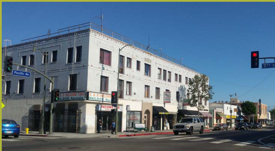
Existing façade conditions on the west side of the 600 (top) and 700 (bottom) blocks of Pacific Avenue
