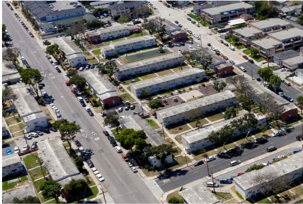
Aerial view of the western part of the Rancho San Pedro public housing development
